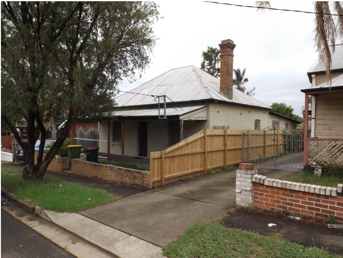
Figure 24 No. 10 Alma Street, recommended for consideration as a new individual heritage item
