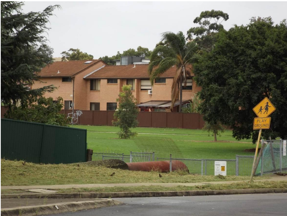
Figure 43 Marsden Street, modern two storey townhouses (viewed from the park)
