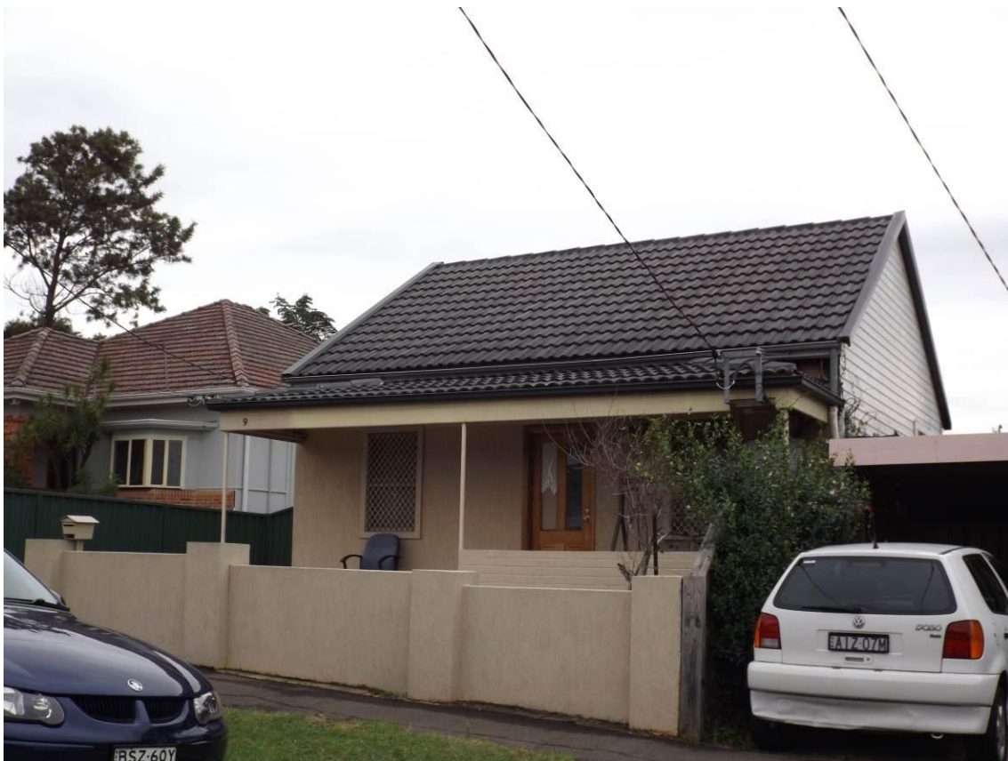
Figure 18 Cottages at No. 9 (top) and 11 (below) Carrington Street
