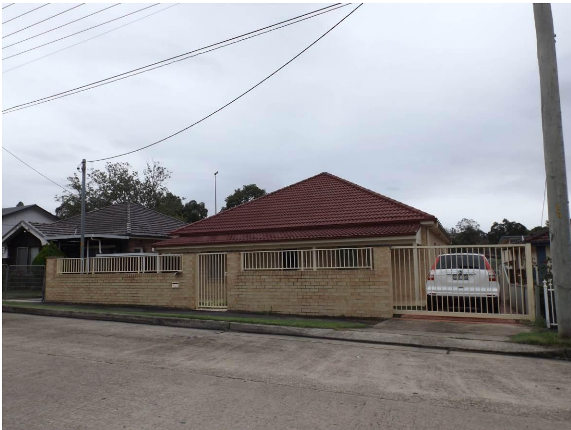
Figure 39 New houses at Nos. 24 (top) and 34 (below) Crimea Street
