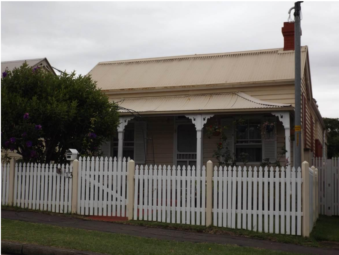
Figure 17 Cottages at No. 15 (top) and 13 (below) Carrington Street
