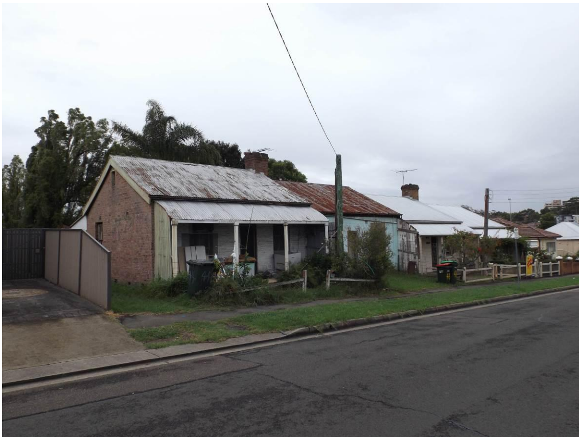
Figure 15 Marsden Street, Nos. 44, 46, 48 and 50 (c. 1880)
