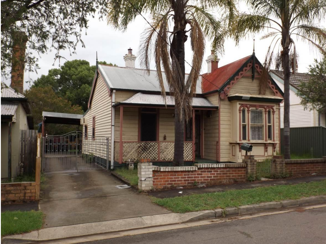
Figure 23 No. 8 Alma Street, recommended for consideration as a new individual heritage item
