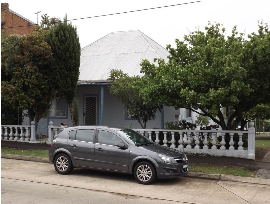
Figure 47 No. 4 Crimea Street, steep roof indicates possible c. 1860-1880s construction
