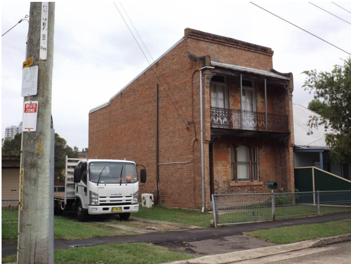
Figure 19 Nos. 8 and 8A (top) and 6 (below) Crimea Street, historical two storey elements in the area
