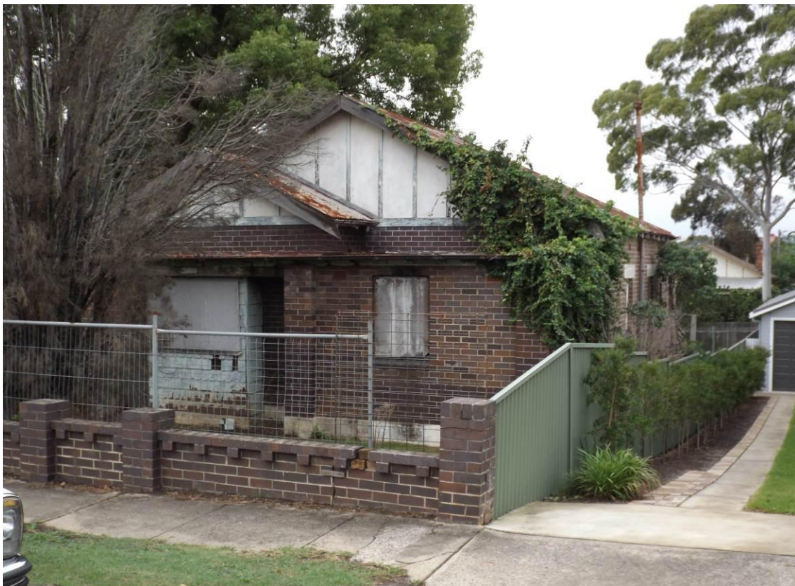
Figure 22 Nos. 13 (top) and 11 (below) Denison Street, recommended for consideration as a new single item (Pair of Bungalows)
