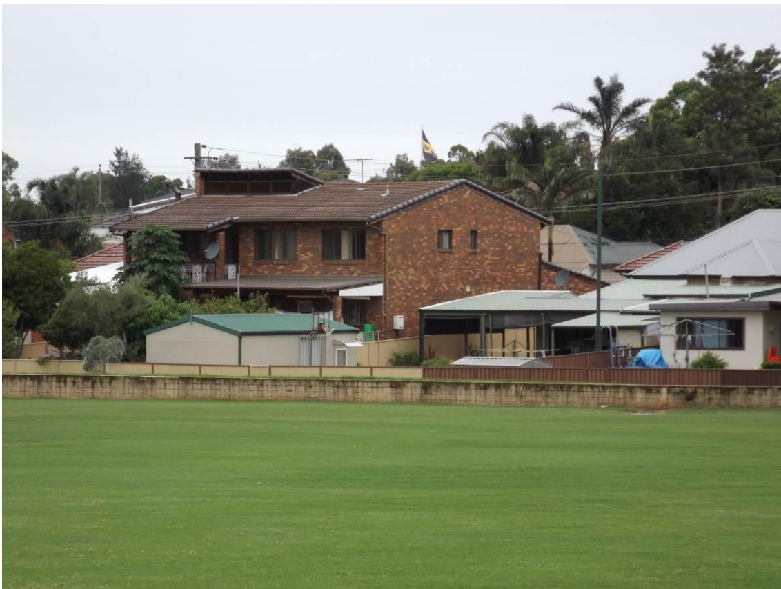
Figure 41 Crimea Street, modern two storey houses (viewed from Glebe Street). See also Figure 42.
